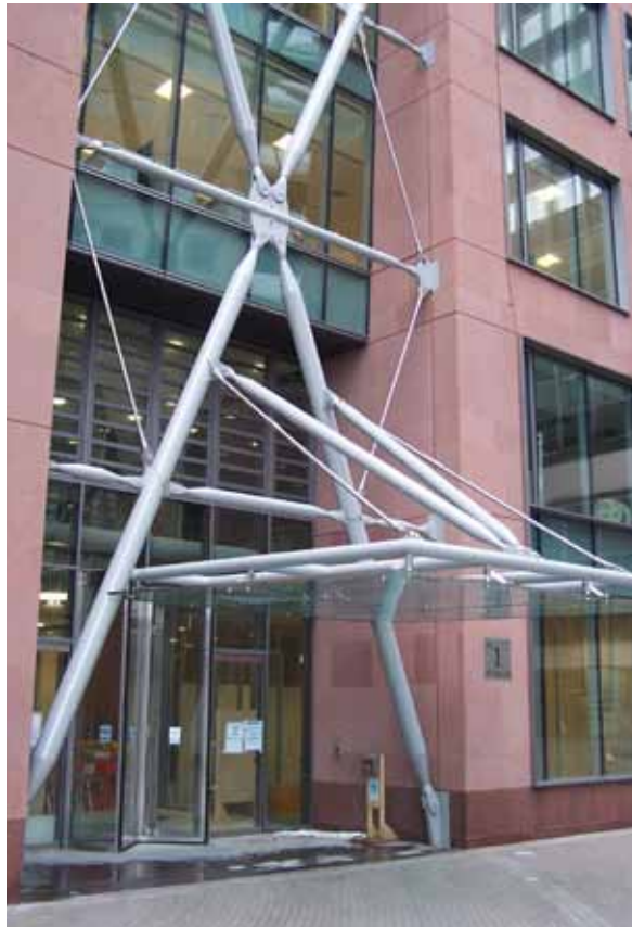
St Paul's Square, Liverpool, UK Architect - RHWL Architects Contractor - Sheperd Construction Engineer - Buro Happold
