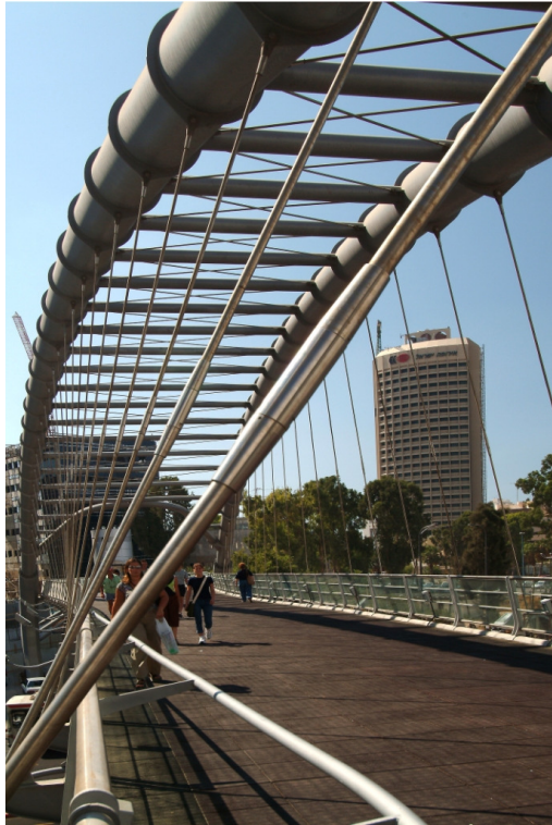
316L Grade Stainless Steel tendons to bridge
